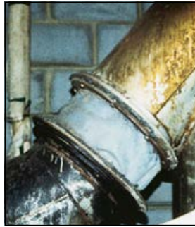
Connectors may be clipped or riveted
