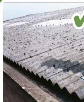
Asbestos cement roofing
