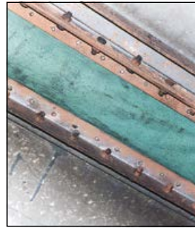
Connectors may be clipped or riveted
