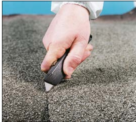
Cut and remove manageable sections
