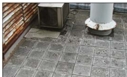
Asbestos cement tiles on a roof
